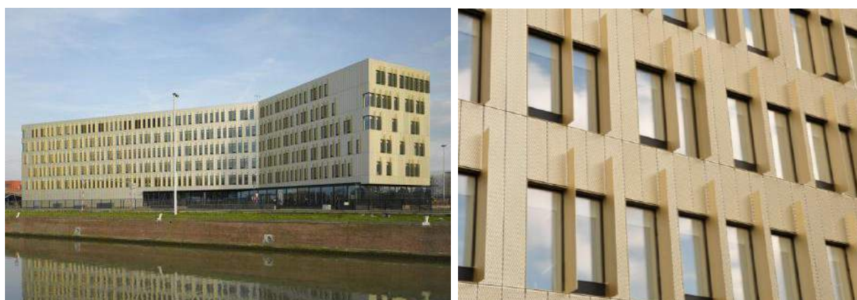
Figure 112 et 113 : Elia Green Building.
